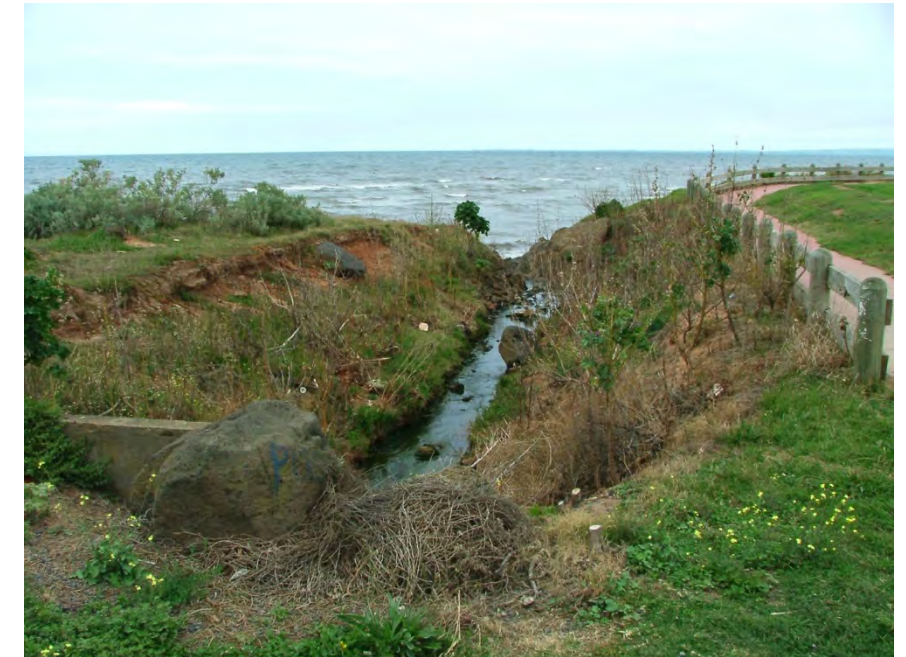
Duncans Road drain outfall
